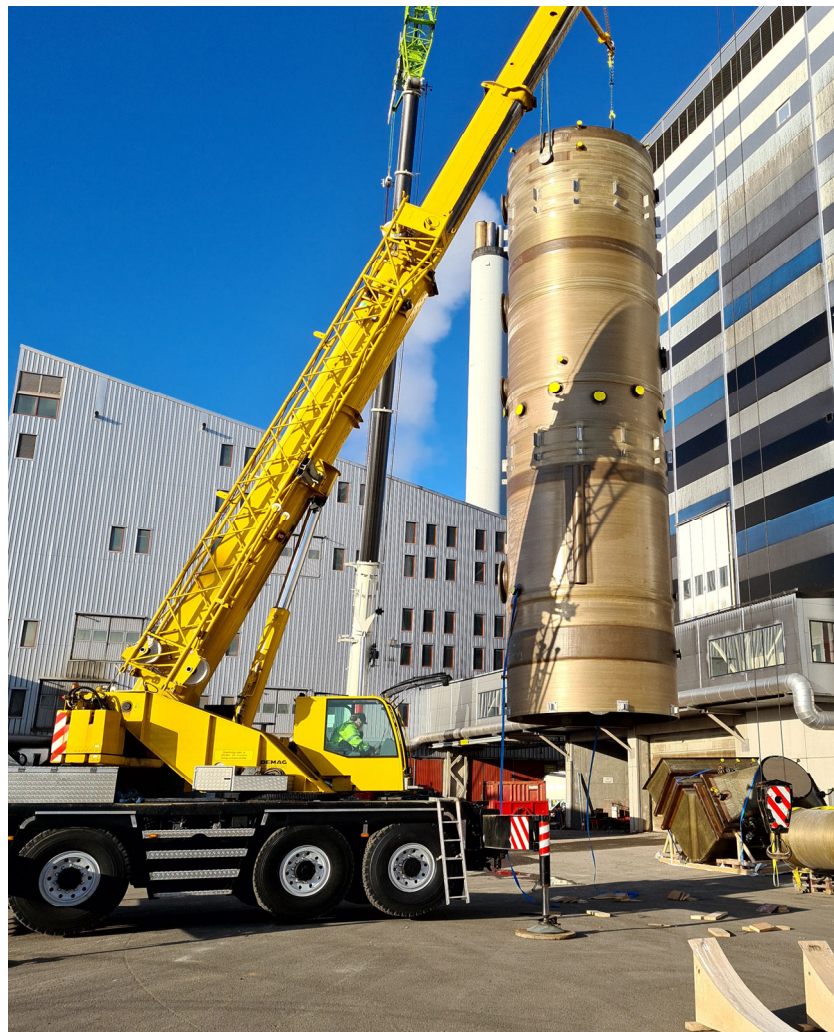
Figure – Lift of scrubber.
