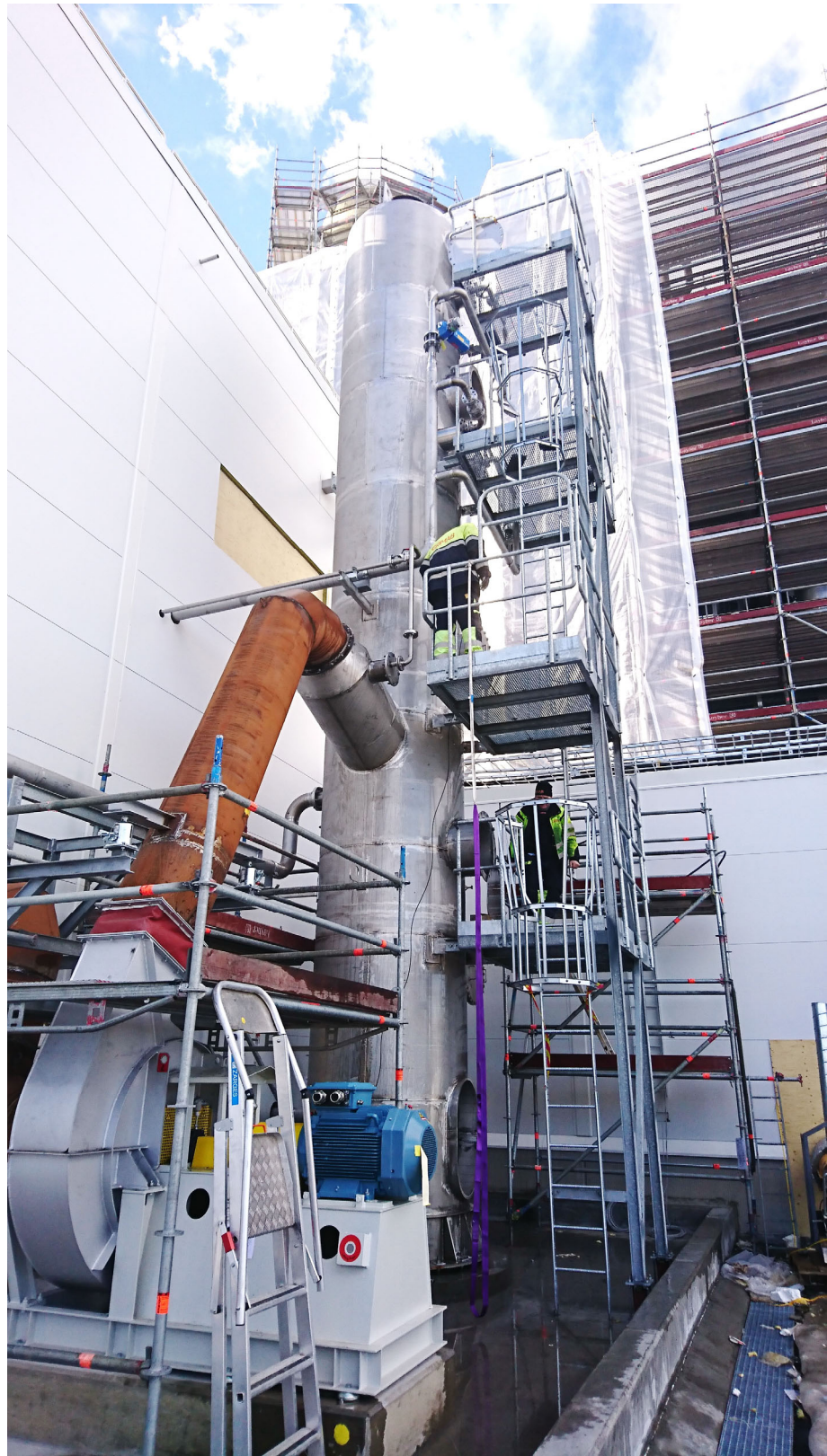
Figure – Scrubber installation for Sunpine AB before thermal insulation.
