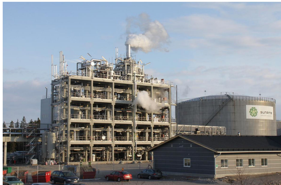
Figure – Sunpine bio diesel refinery.
