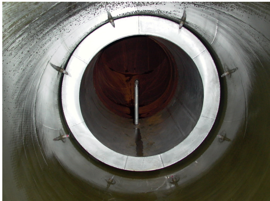
Figure – Interior of quench for combined scrubber/ wet ESP for Perstorp Specialty Chemicals.
