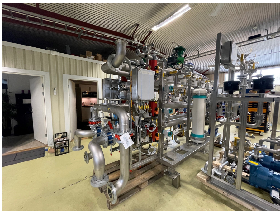
Figure – Manufacturing of ultra-filter skid.
