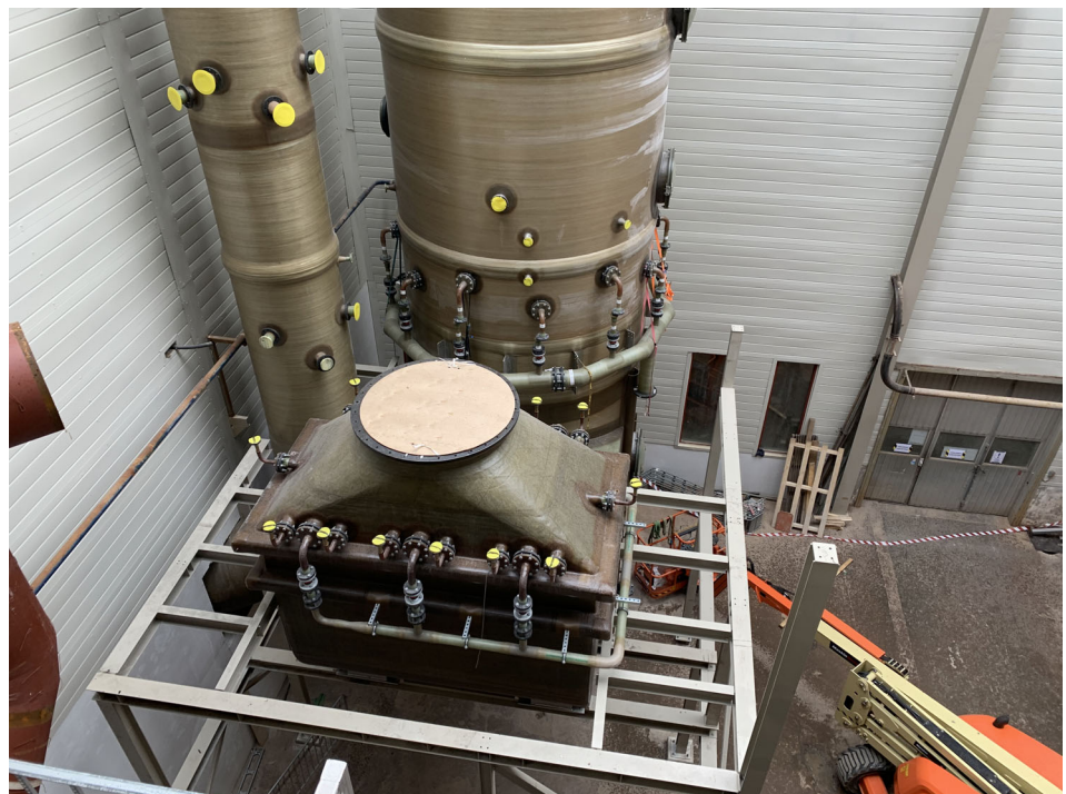
Figure – Installation of scrubber tower in Lidköping.
